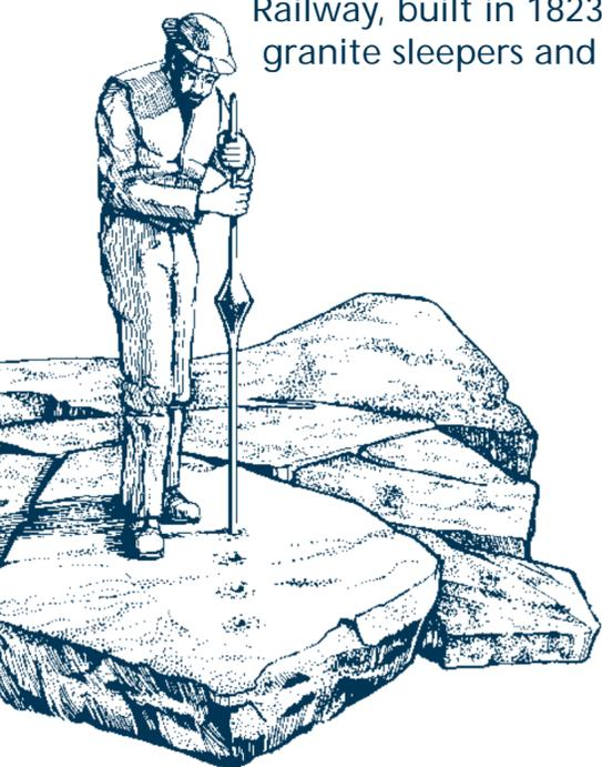
1 Using a 'jumper' (a weighted, one-person operated drill), a line of holes was drilled approximately four inches deep and six inches apart.
