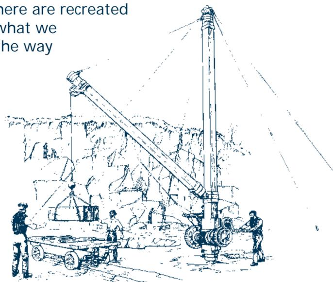
3 The large blocks of granite were lifted onto flat-topped trucks by means of a derrick (remains of the derrick illustrated can be seen at Haytor Quarry). This was operated by hand and had two gear trains. The whole unit pivoted on a metal bearing sunk into the granite (still visible), the top being held vertical by metal rods which were joined to allow flexing under the load.
